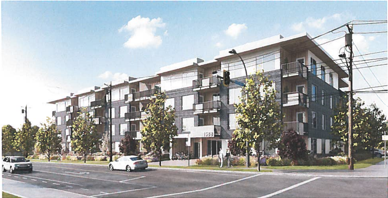
Figure 3: Corner View at North Dairy Road & Wordsworth Street (from plans by Low Hammond Rowe Architects)
